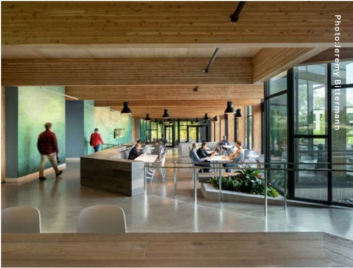
First Tech Federal Credit Union includes a 12x32-ft grid with 5-1/2-in. CLT panels spanning 12 ft between glulam beams.
