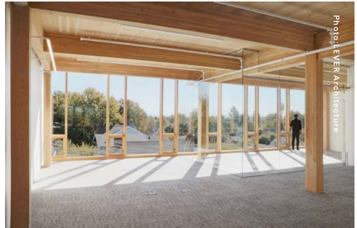
Albina Yard is built on a 20×20-foot grid with one intermediate beam in each bay and 3-ply CLT panels spanning 10 feet between glulam beams
